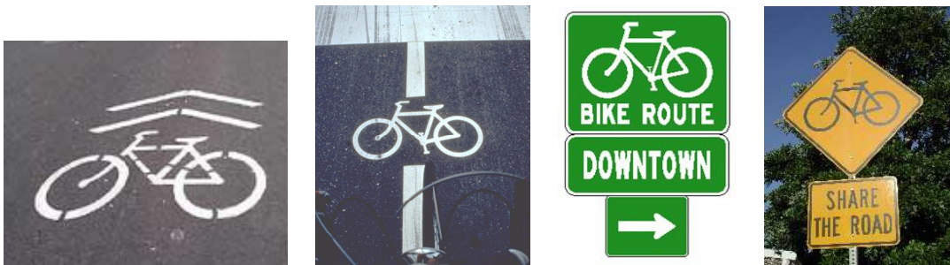
Figure 3 – Pavement Markings and Signage: “Sharrows” – indicates proper bike position in the presence of on-road parking; on-road traffic signal actuation for bicycles; Bike Route signage with wayfinding; Share the Road signage.
